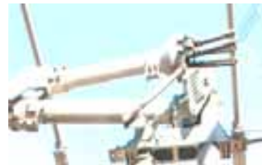
GW16 is for vertical disconnect switch.
