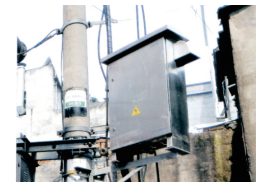
Installed capacity of a certain station area in Henan: 100 kVar
