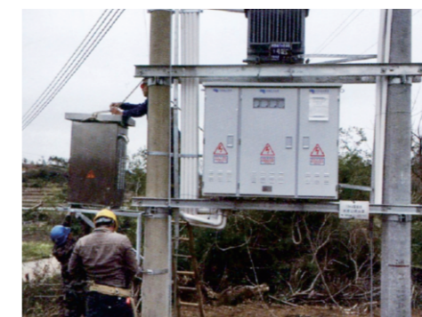
Installed capacity of a certain station area in Guangdong: 100 kVar
