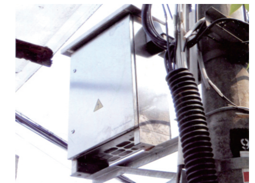
Installed capacity of a certain station area in Anhui: 100 kVar
